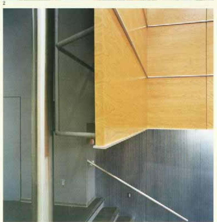
upper walls, refinished in aluminum-splined oak-faced panels, wrap the stage, forming a proscenium (4). Over the stage, expanded-metal fabric conceals speakers and theater lights (2).
